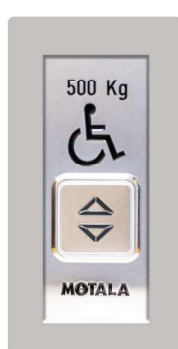
Floor Buttons In The Wall
